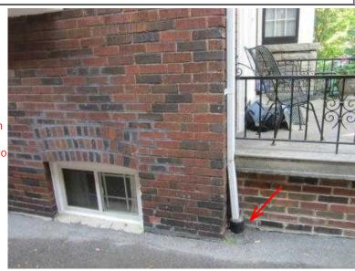
20. Marginal Leader/Extension: Missing: Extend downspouts to move water away from foundation
