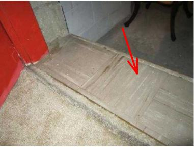
5. Acceptable Floor Drain: Surface drain
