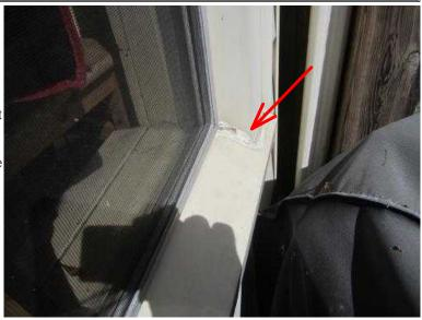
8. Acceptable Window Sills Stone - jointed: Joints in sills frequently crack and allow moisture to penetrate - monitor regularly
