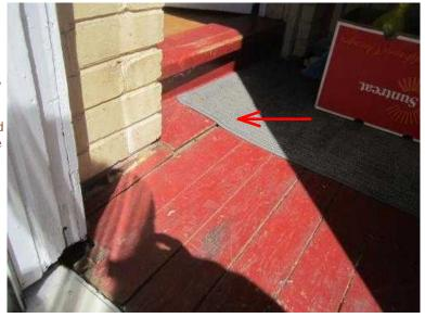
4. Not Inspected Foundation: Not visible: Floor settled - foundation is likely lacking, as is common in these older add-on mudrooms.
