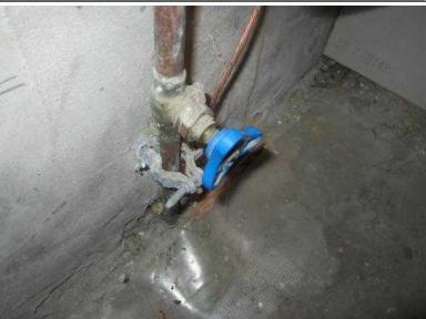
4. Acceptable, Improve Water Lines: Copper: Note that the exterior water shutoff at the rear is not
